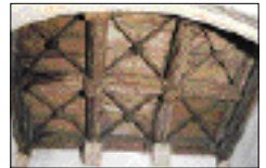
Godolphin Chapel ceiling.
