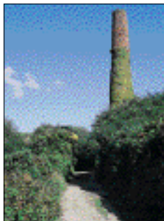
Watson's Shaft chimney stack.
