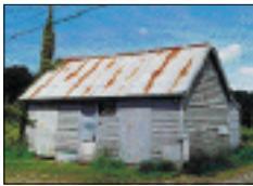
Men's Institute before demolition in 2001.
