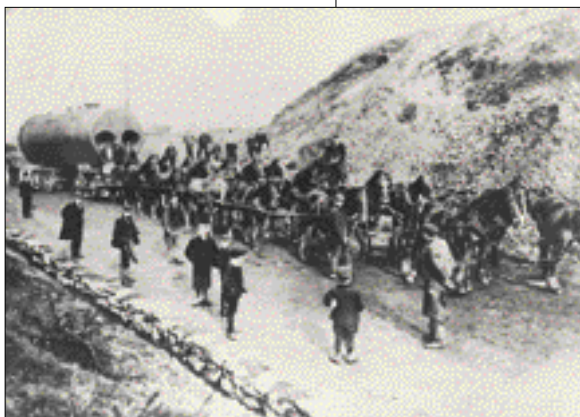
A team of horses pulling a mine boiler from Harveys of Hayle to Wheal Vor Mine in 1906. The horses were owned by Mr Will Tyacke of Carleen and driven by Harry Meagor.
