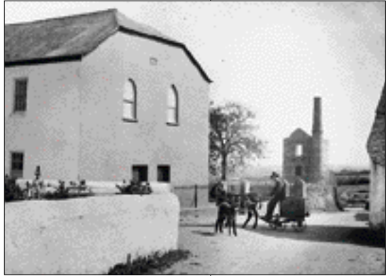
The water carrier at Carleen with the Methodist Church on the left. In the distance is Flat Rod Shaft engine house of Carleen Mine, which was demolished in 1948.
