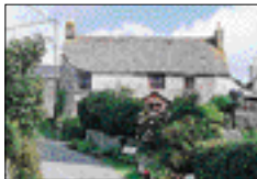
Old cottage at Germoe.
